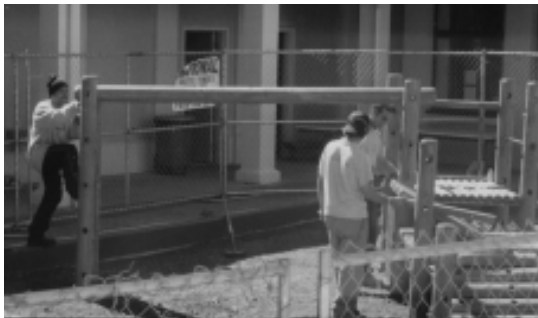
Tearing out the old equipment
